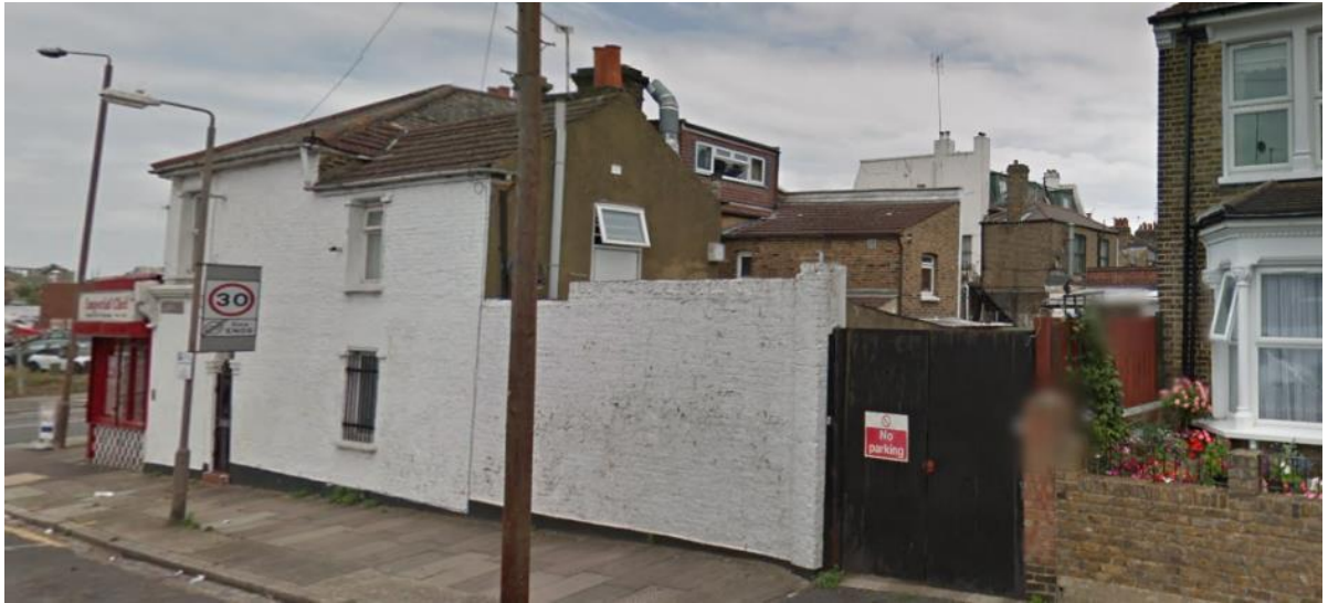
Plate 8: Facing north east
